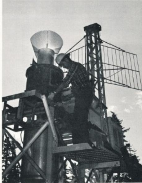
Fig. 11 -- Pacific Gas & Electric Company ground-based silver iodide generator.
